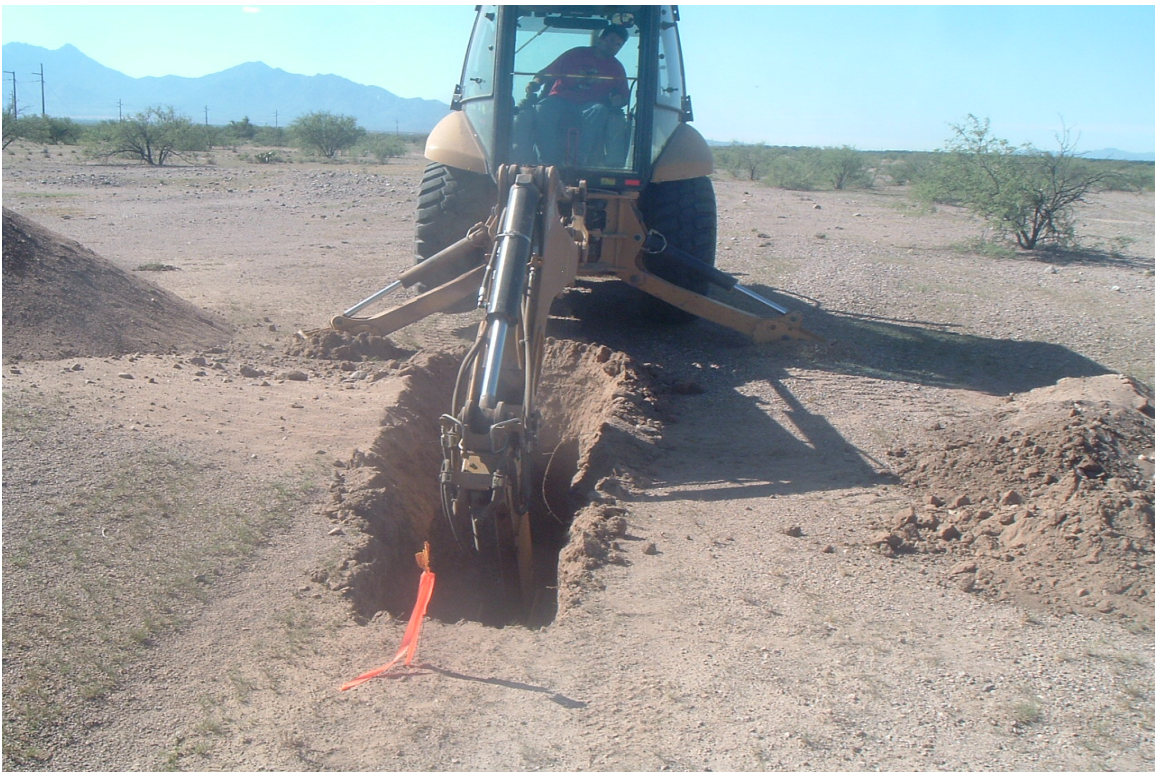
Figure 4-10. Backhoe Test Pit
